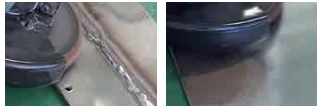
Removing blue weld discoloration Removing Rust
